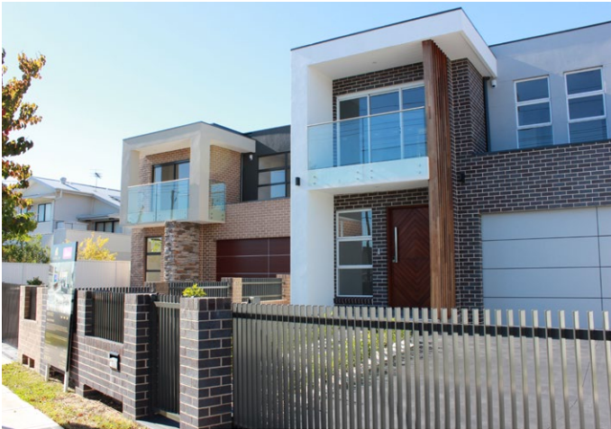
Dual occupation project homes in Canley Vale
