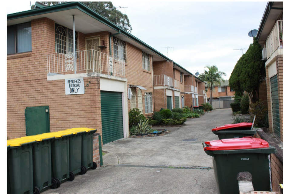
Typical gun-barrel housing that has a poor street interface and limited privacy and amenity for residents-Carramar
